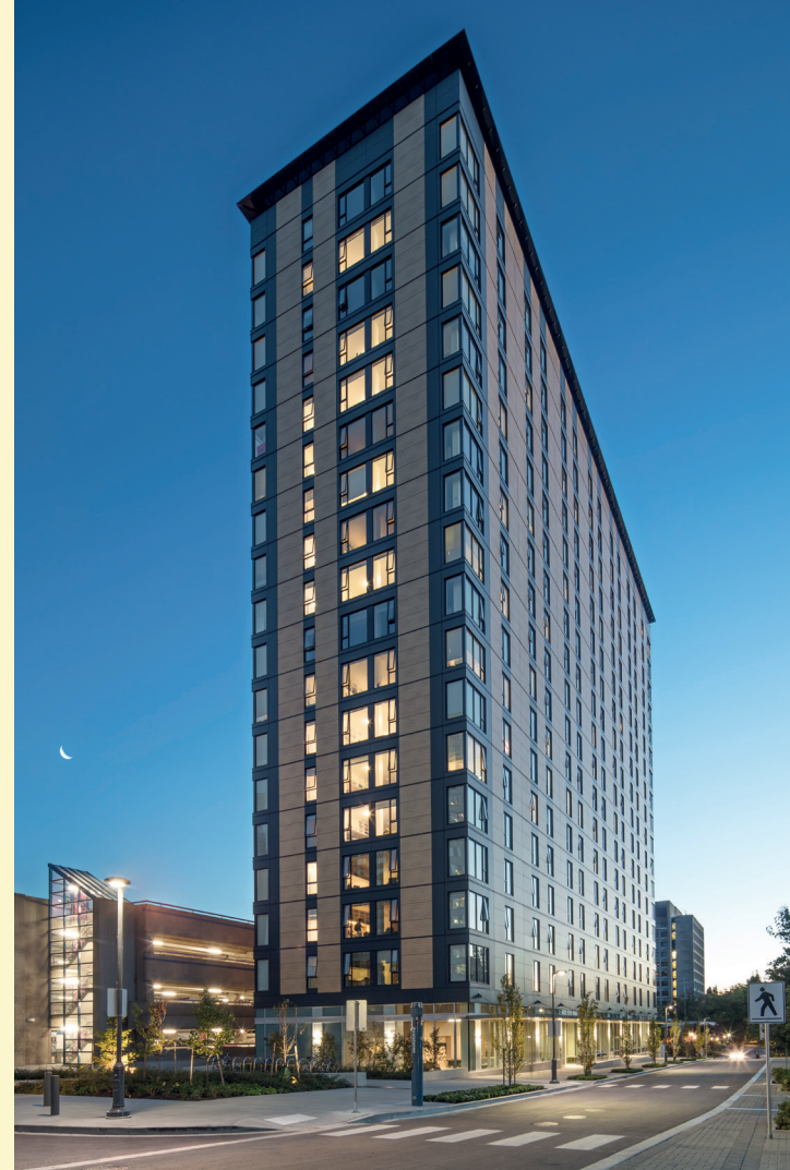
↑ Brock Commons Tallwood House is an 18-storey student residence at the Point Grey Campus of the University of British Columbia in Canada. At the time it was opened in 2017, it was the tallest mass timber structure in the world.
