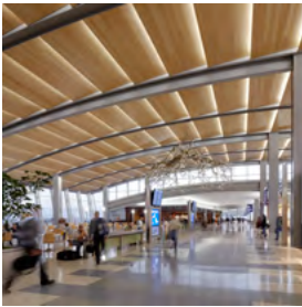
Timber board products using soya-based glue by Columbia Forest Products, top, and applied as ceiling panels at Sacramento Airport, bottom. Modifications to the soy protein glue base were modelled on marine proteins found in blue mussels, to improve adhesion strength and durability.
