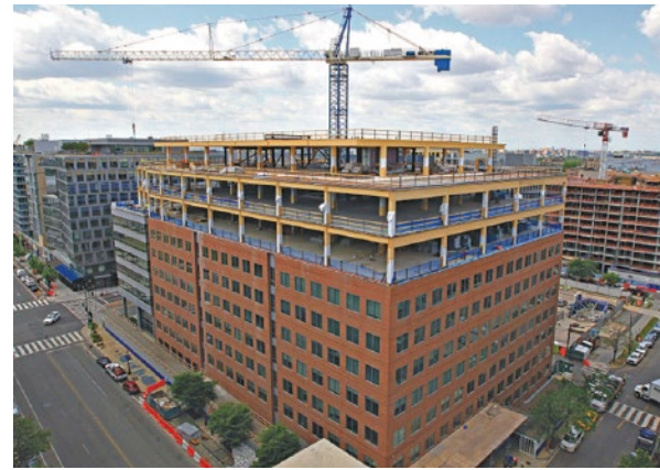
Wood's lighter weight makes it the ideal material for 'building-on-top' of existing buildings in urban areas allowing cities to grow without building on more countryside
